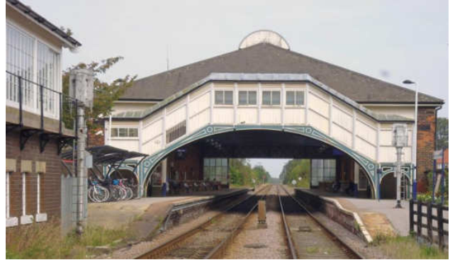
Note the grill on the left to allow the signal man to see all the down-platform.
